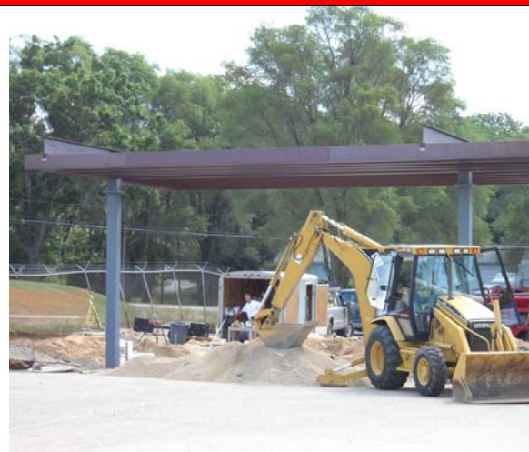
Gas Pump Canopy
