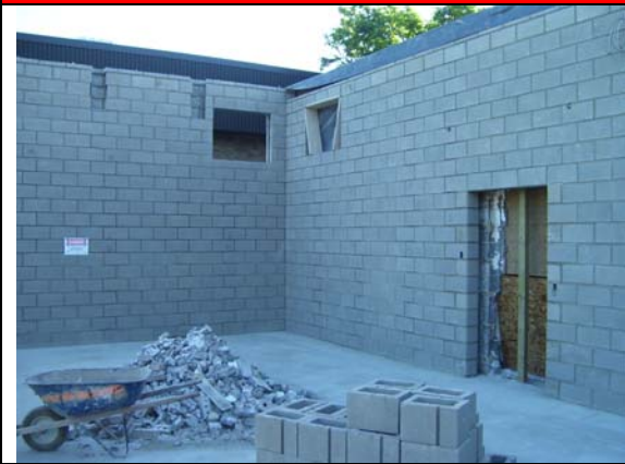
Storage Addition Masonry Walls
