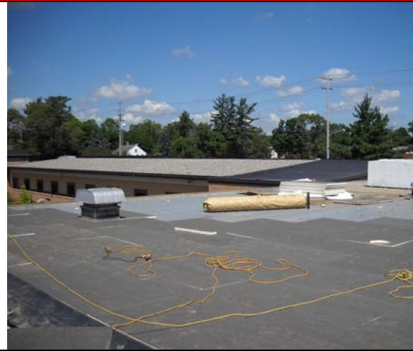
New Roof Membrane
