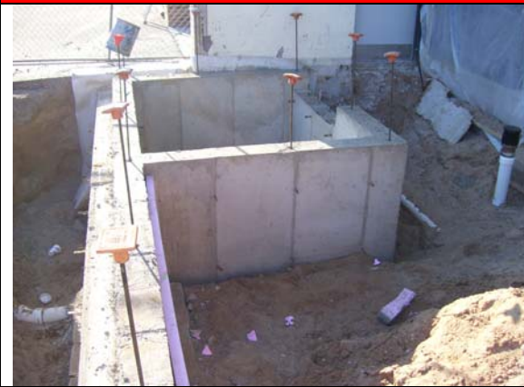
Stairwell/Elevator Foundation Walls
