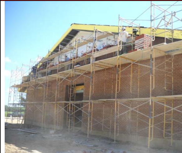
Finishing up Brick on Gable End
