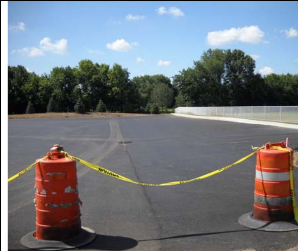
South Site Parking Lot
