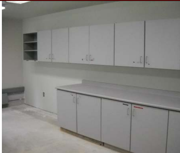
Reinstalled Millwork
