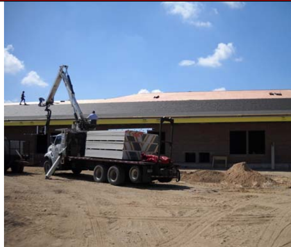
Delivering Drywall for Ceilings
