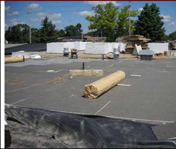
New Roof Membrane
